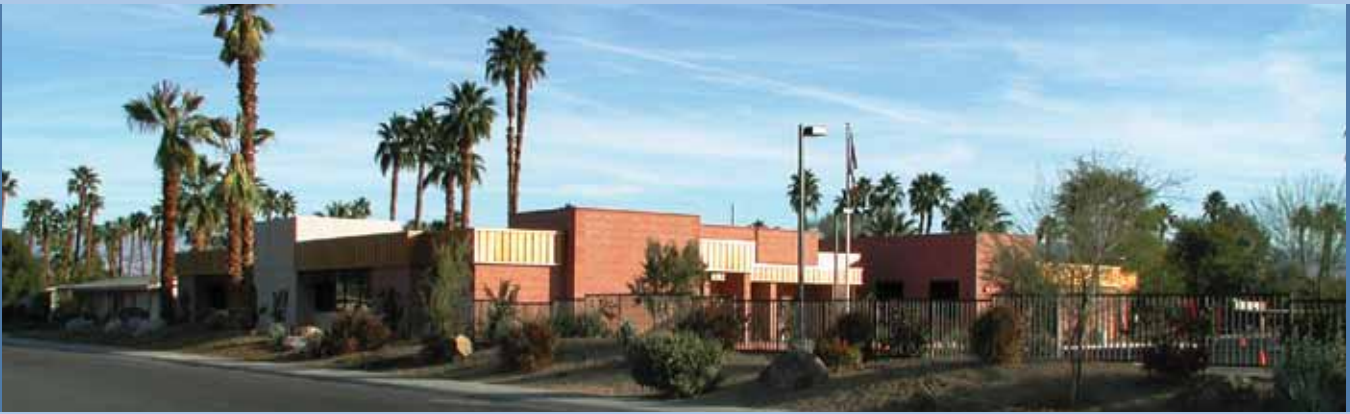
Sacred Heart – Administrative Office and Classroom Addition
