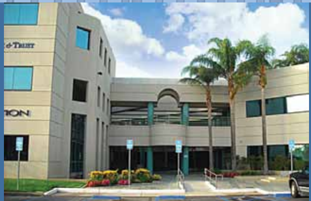
Palmbrook Corporate Center – Multiple Tenant Improvements
