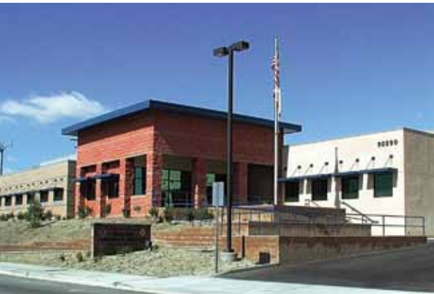
Cabazon Sheriff Station – New Design/Build facility
