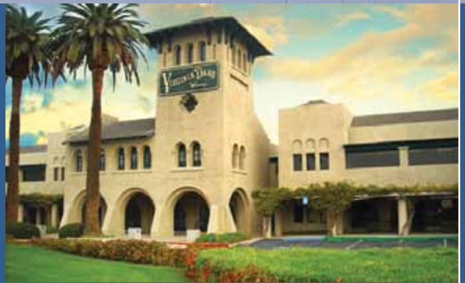
Virginia Dare Tower – Multiple Tenant Improvements
