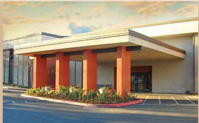
Redlands Medical Center - Tenant Improvements
